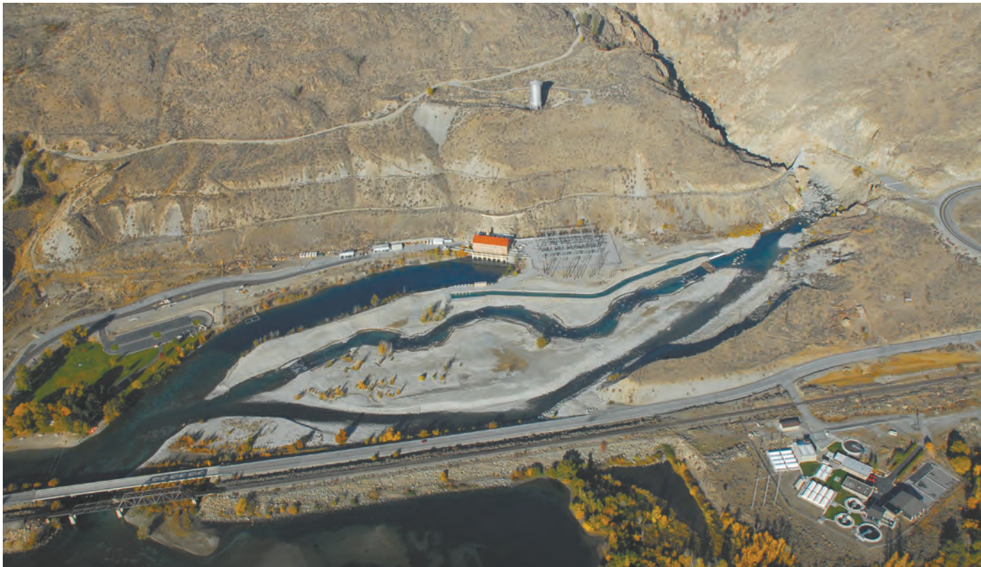
Aerial photo shows new channel designed to attract fish (undulating channel in center of light gray area).
